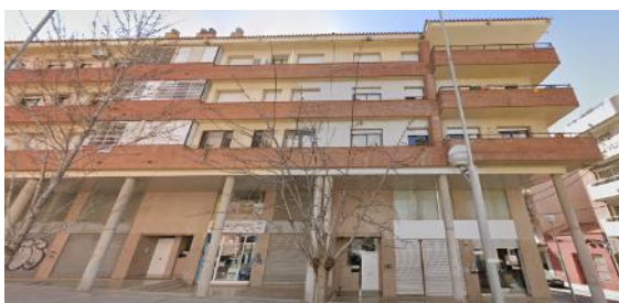
Residential (Terrassa, Spain)
