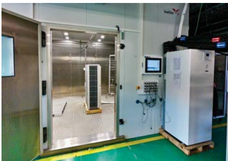
Heat pump in our testing lab
