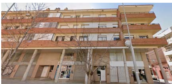
Residential (Terrassa, Spain)
