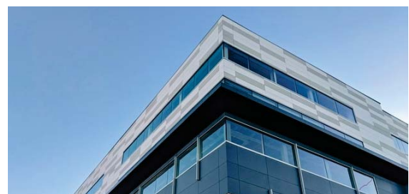
Office buildings (Manresa, Spain)
