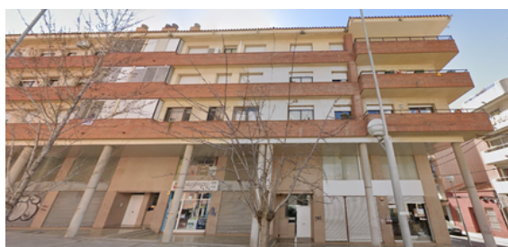
Residential (Terrassa, Spain)
